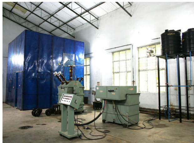
Fig. 1 Artificial pollution experimental facility
